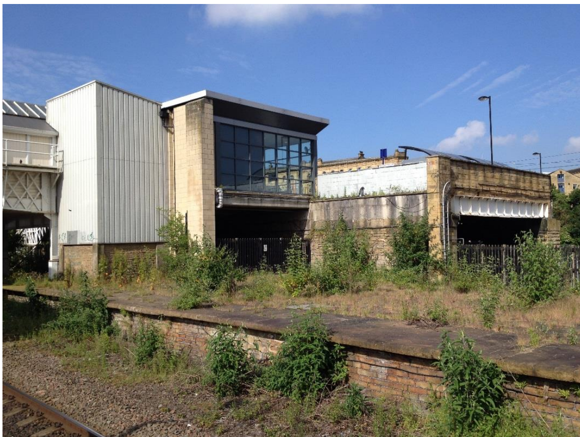
Photograph 1.6 – Halifax Rail Station Buildings
