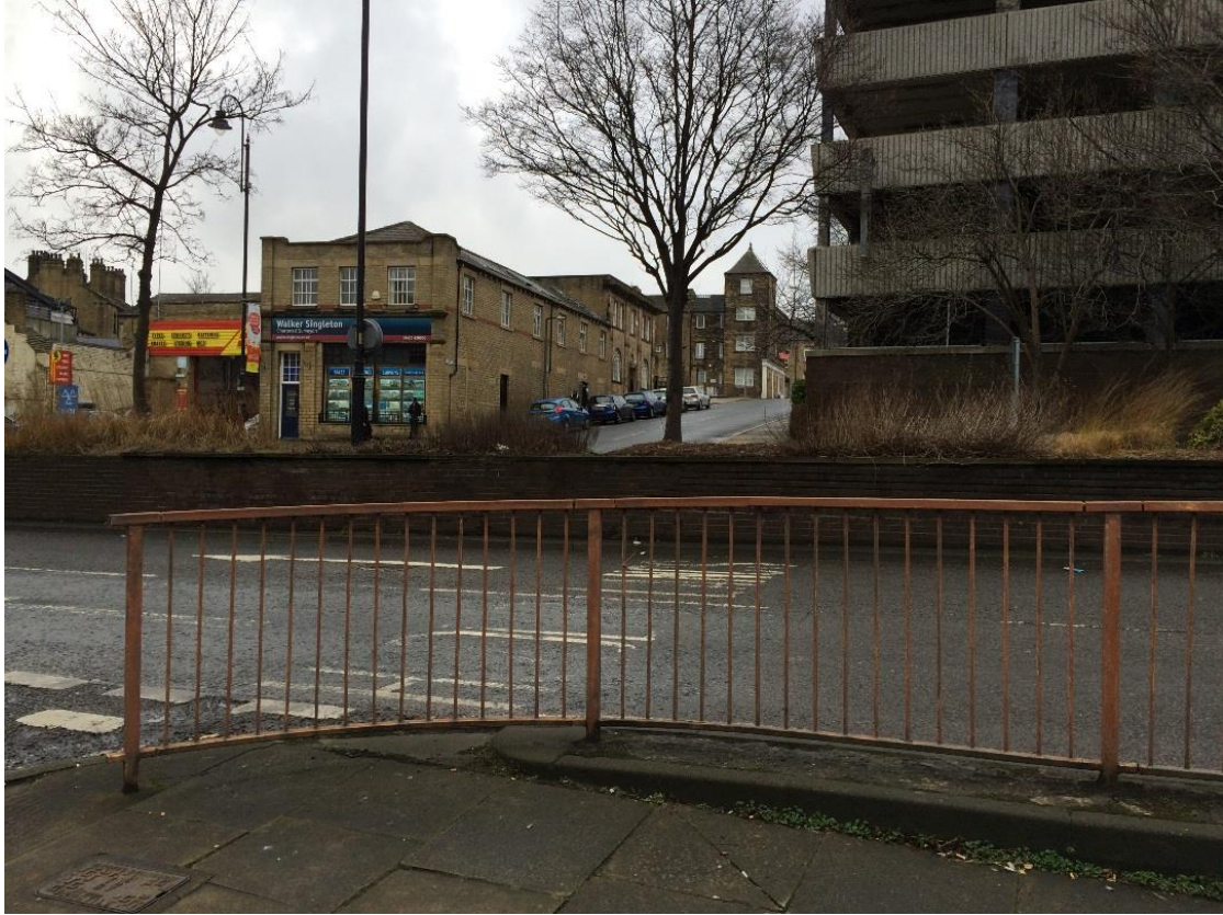
Photograph 1.3 – Pedestrian Guardrail at Town Centre Junctions
